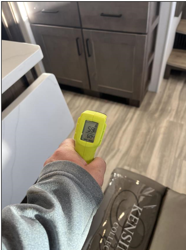
Living area no air discharge
