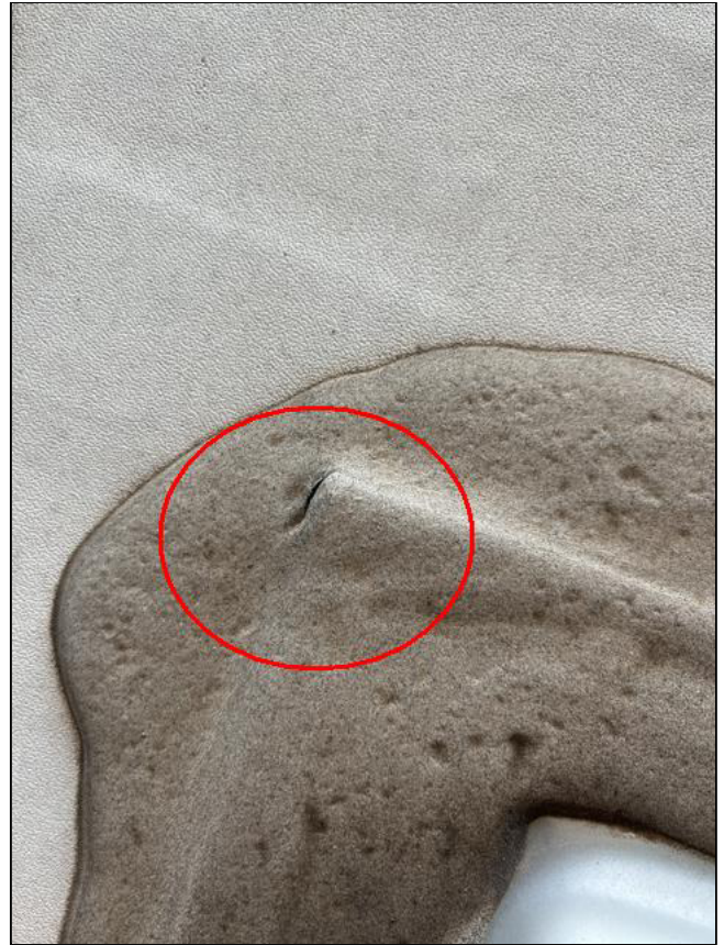
Sealant Crack
