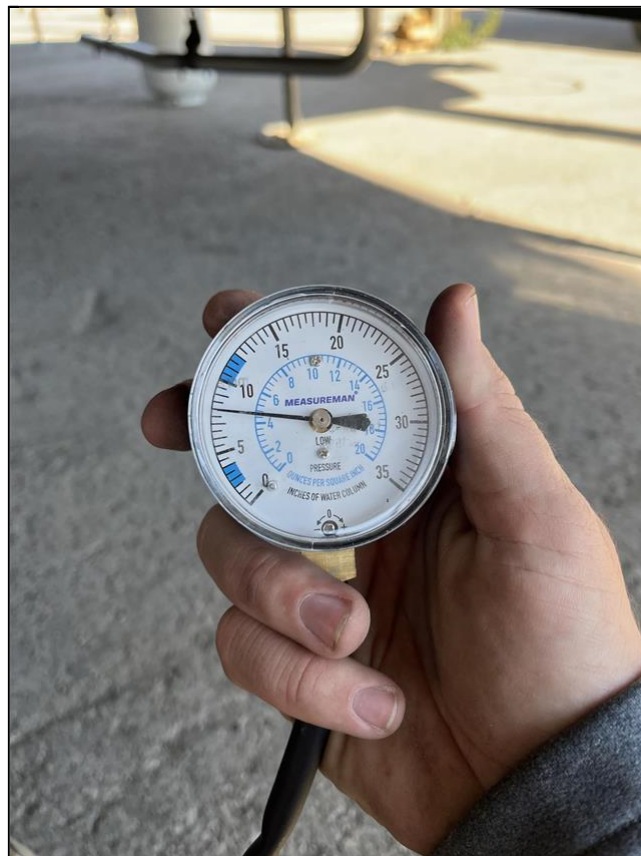
LP Leak Test
