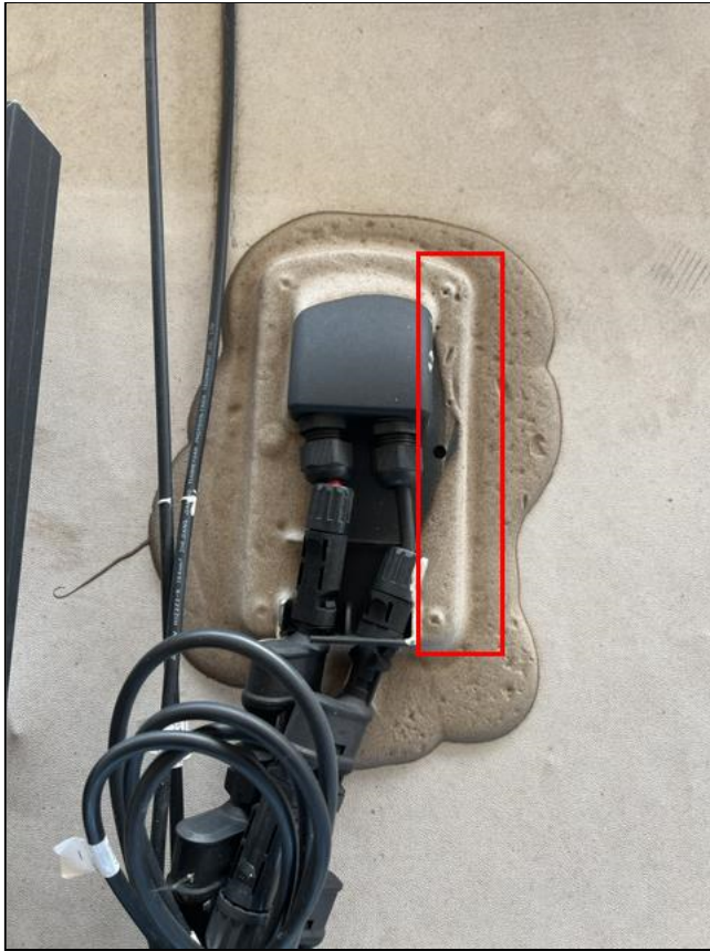
Solar Roof Penetration
