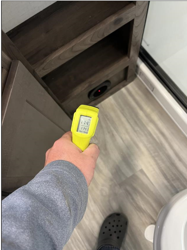
Bathroom Warm Air Discharge
